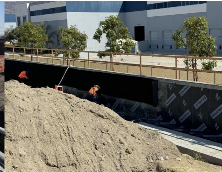
East Retaining Wall Waterproofing
