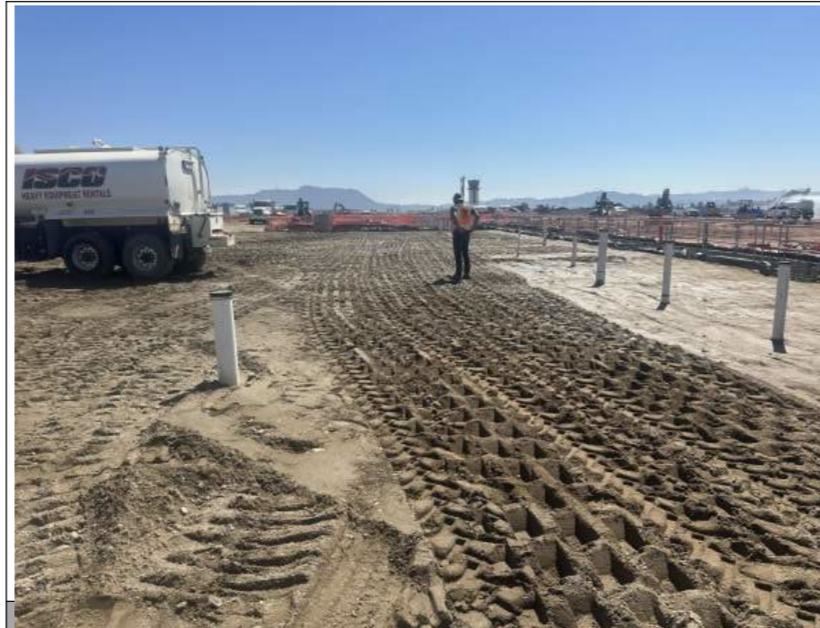
Area C Backfill
