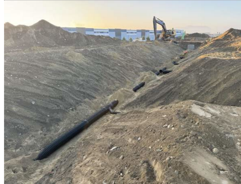
Storm Drain Line Install
