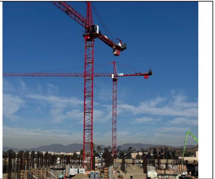
Parking Garage Cranes
