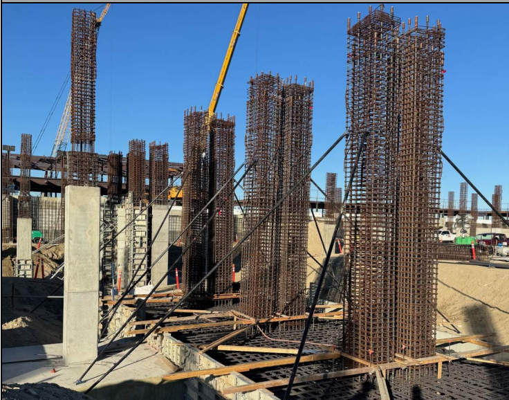
Parking Garage Foundations
