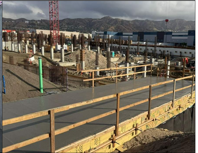
Tunnel Lid Concrete
