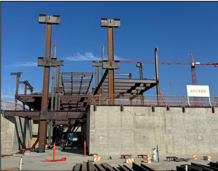
Terminal Area C Steel Erection
