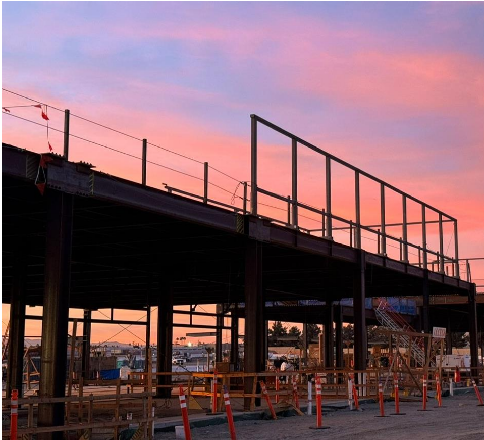
Terminal Area A and B Steel
