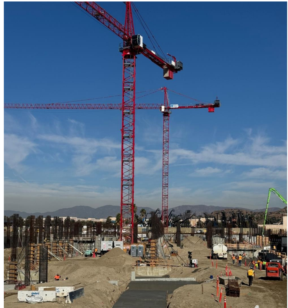
Parking Garage Cranes
