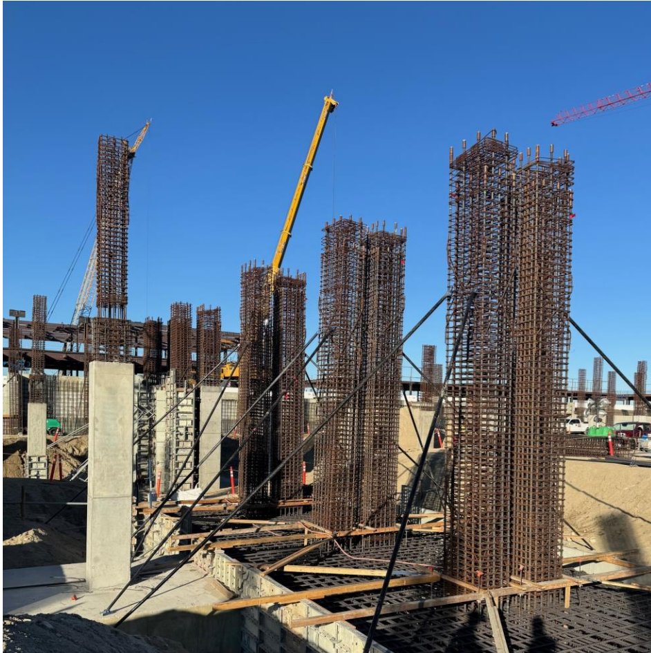
Terminal Area C Steel Erection
