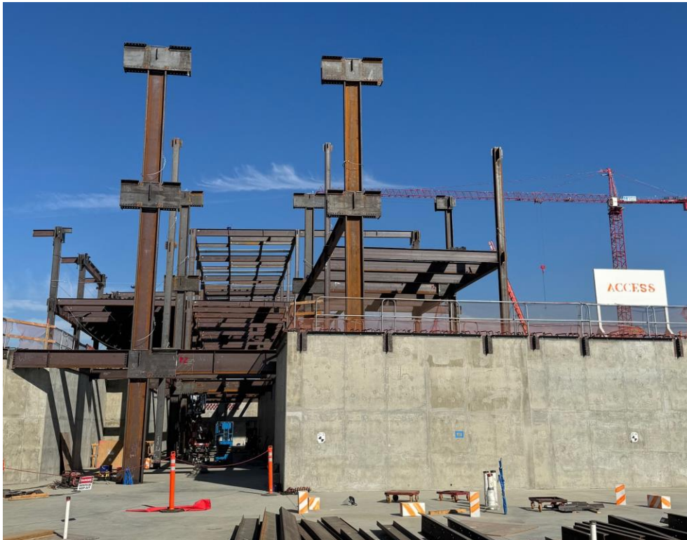
Terminal Area C Steel Erection
