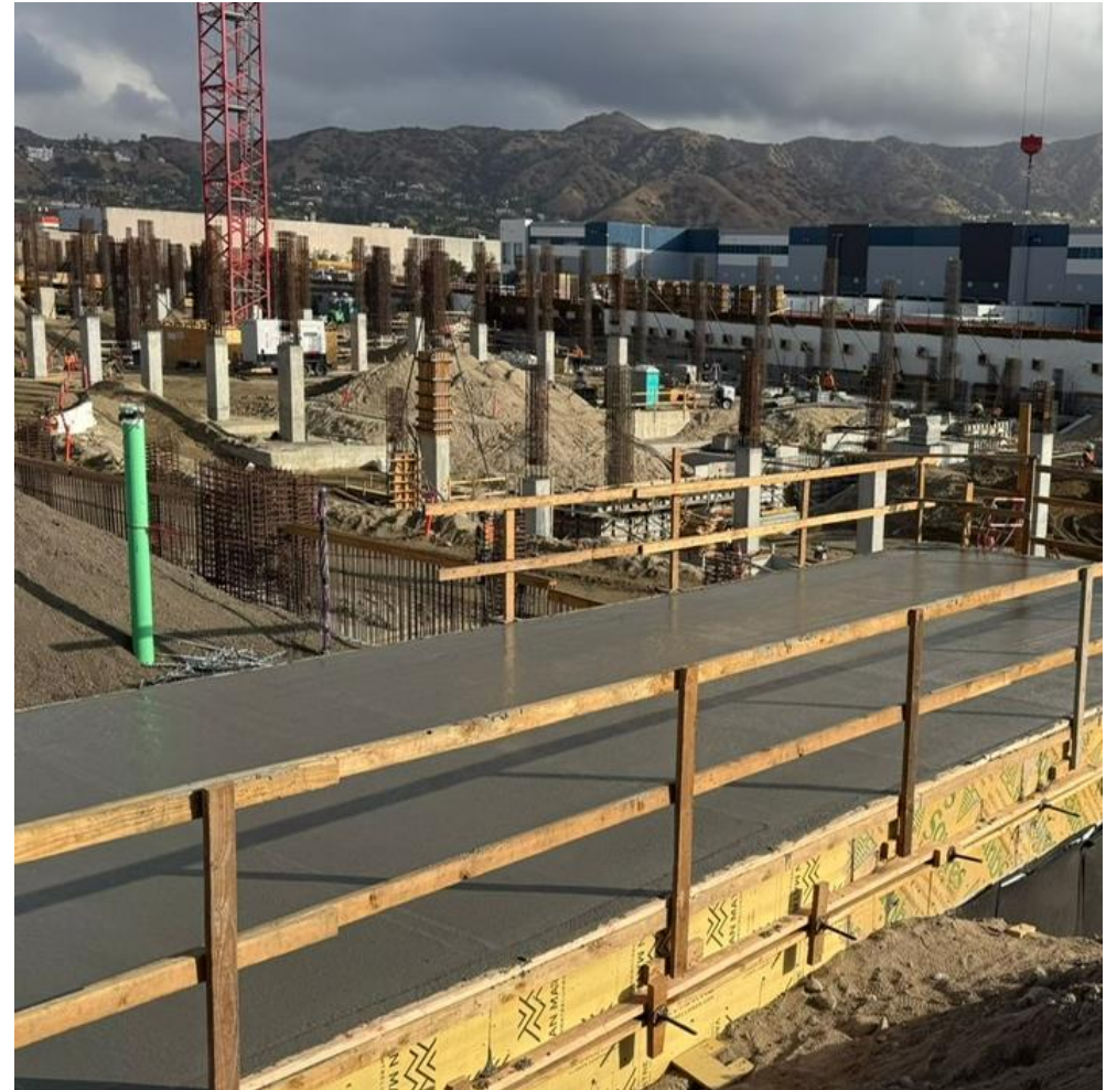
Tunnel Lid Concrete
