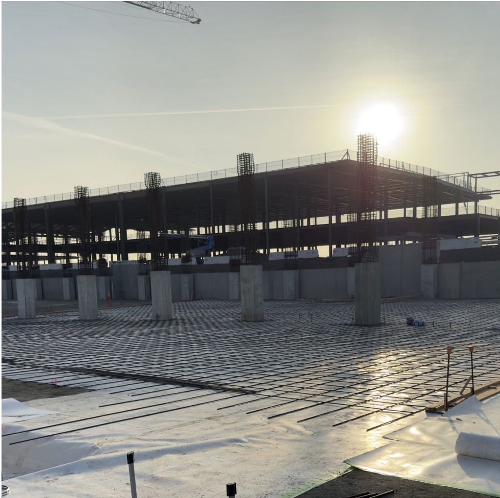
Parking Garage Rebar & Terminal Steel
