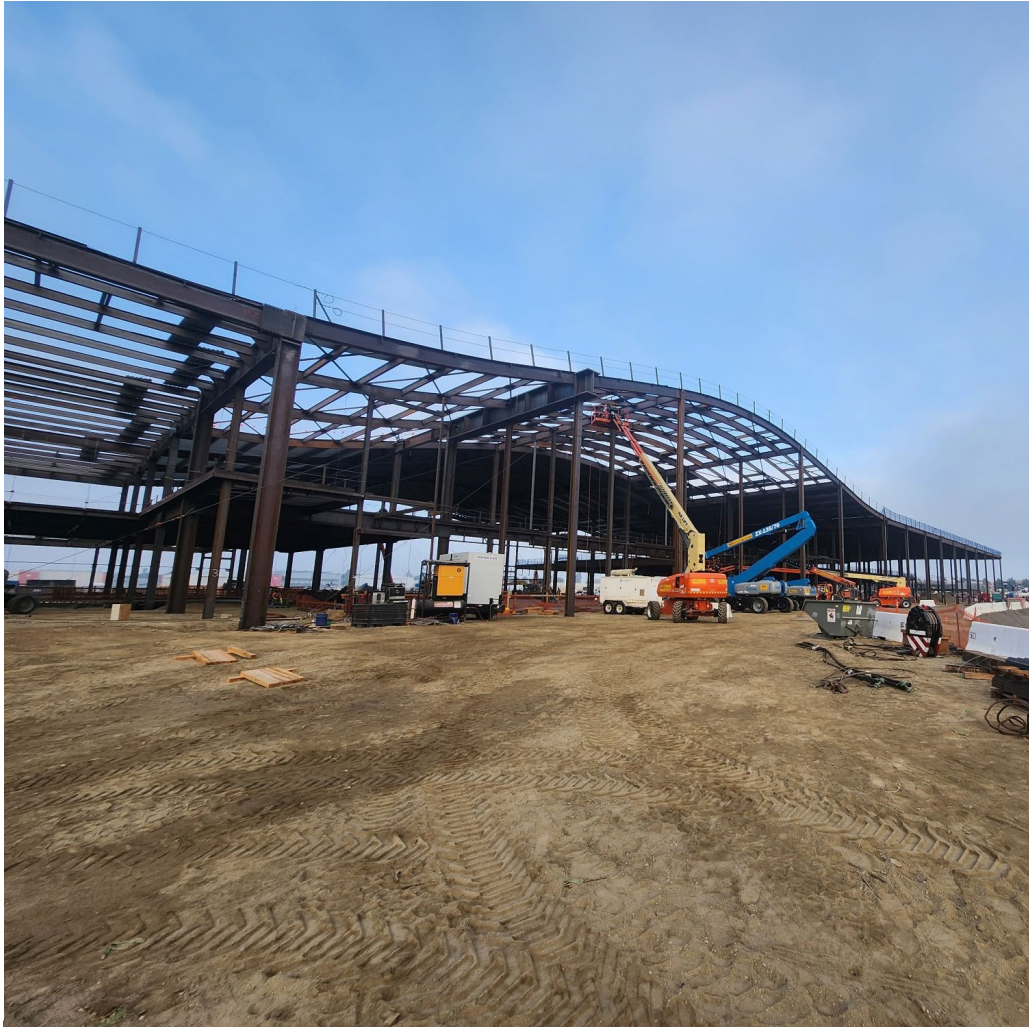
Terminal Area C Steel Erection
