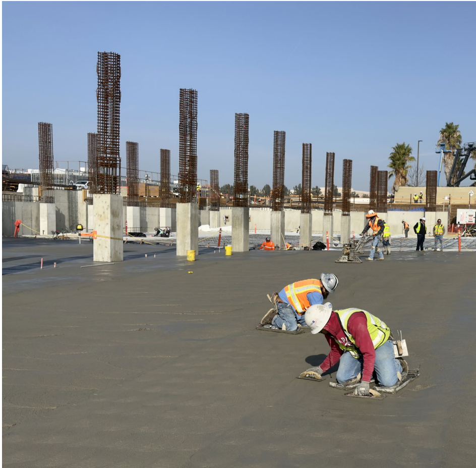
Parking Garage Slab Finishing
