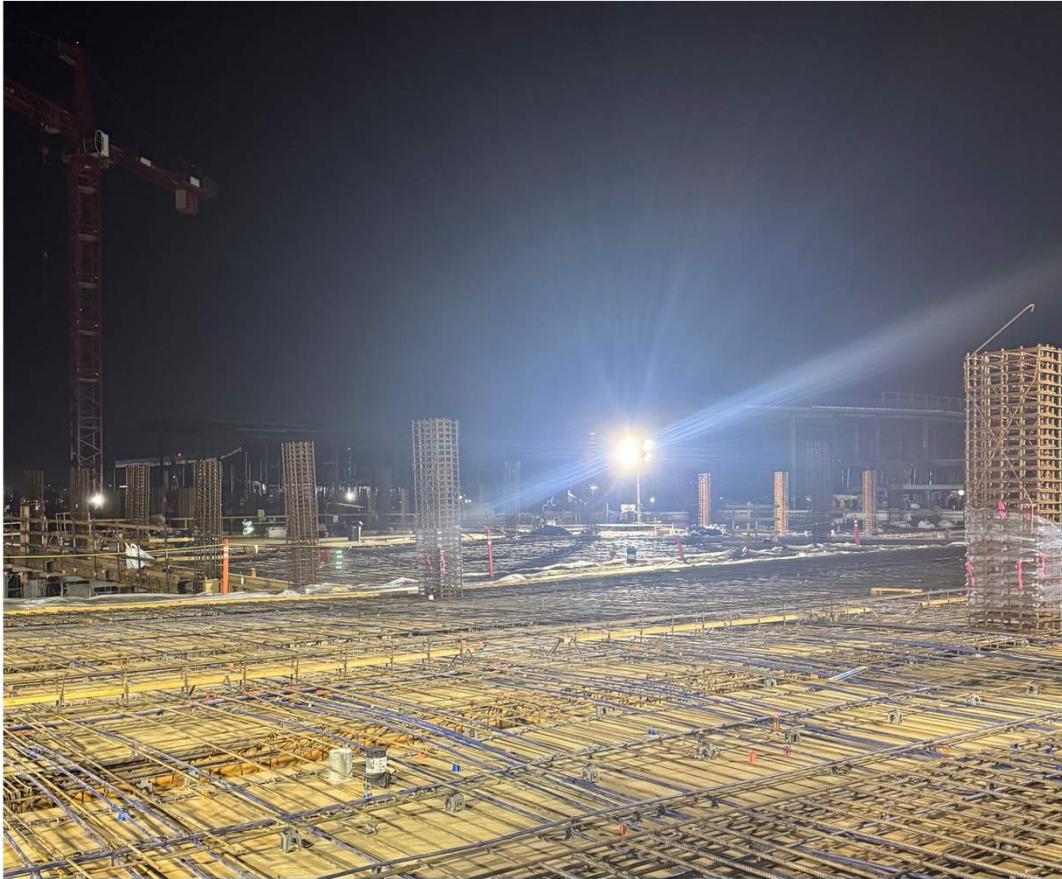
Parking Garage Elevated Deck
