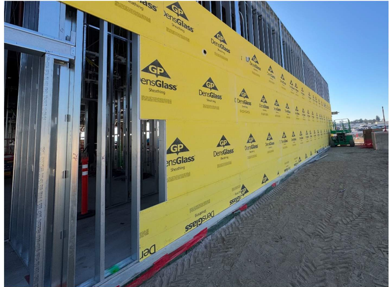
Terminal Exterior Framing
