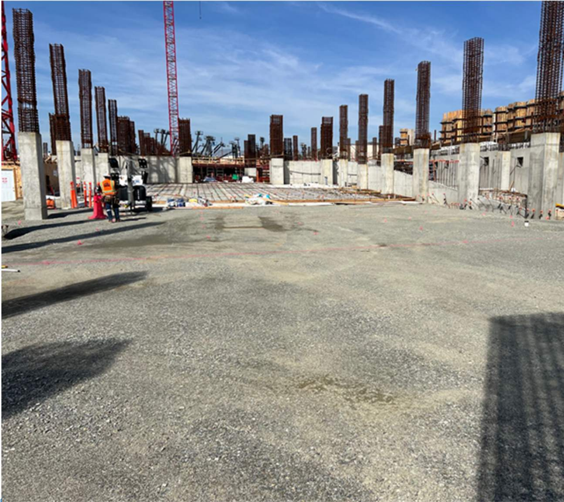
Parking Garage Base Installation
