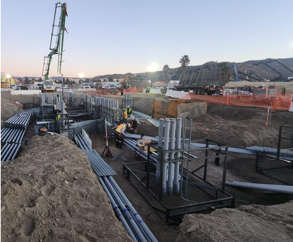
Electrical Ductbank Installation
