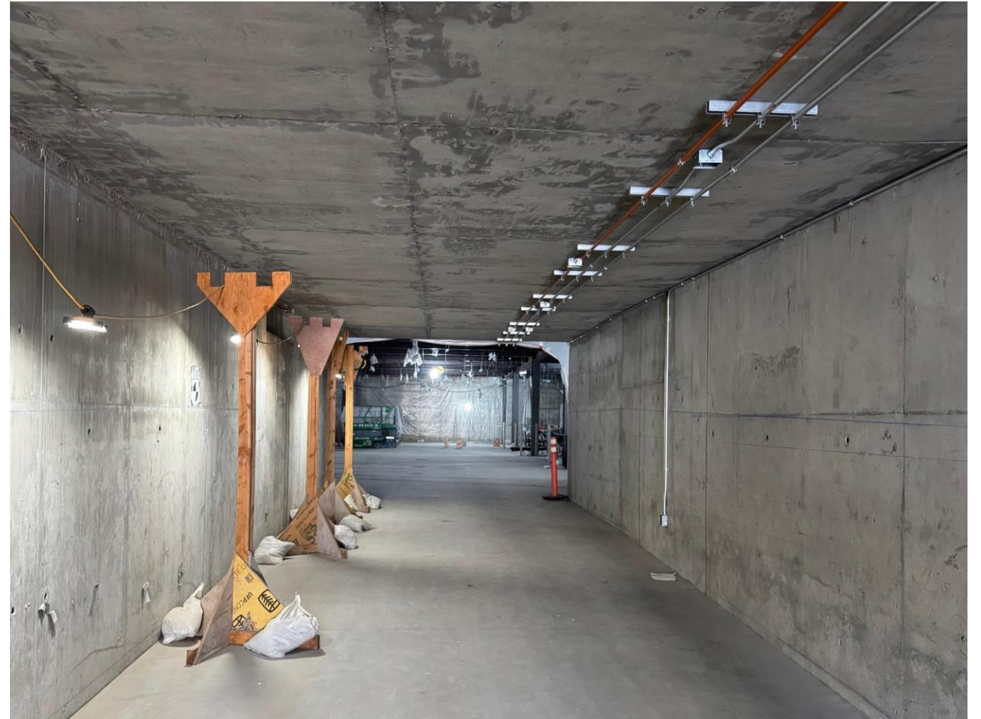
Terminal to Garage Tunnel
