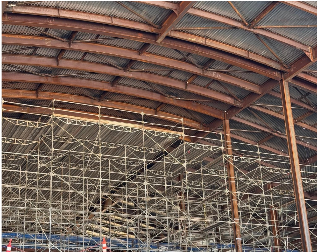
Terminal Scaffolding Install
