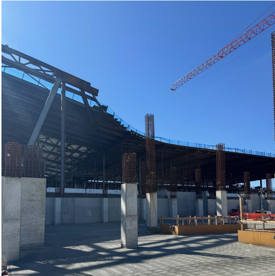
Parking Garage Slab on Grade
