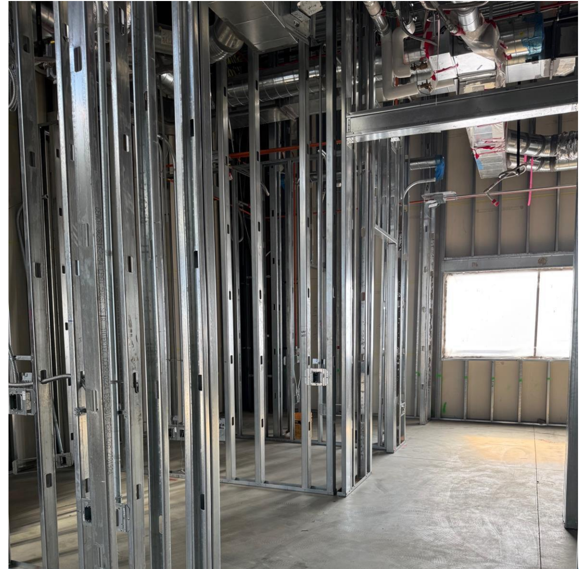
Terminal Interior Framing
