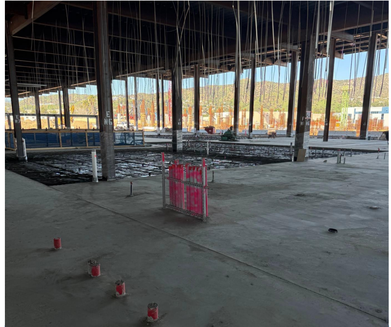
Terminal Slab on Grade
