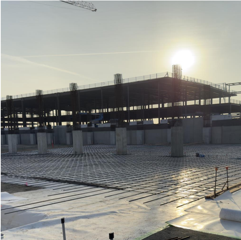
Parking Garage Rebar & Terminal Steel
