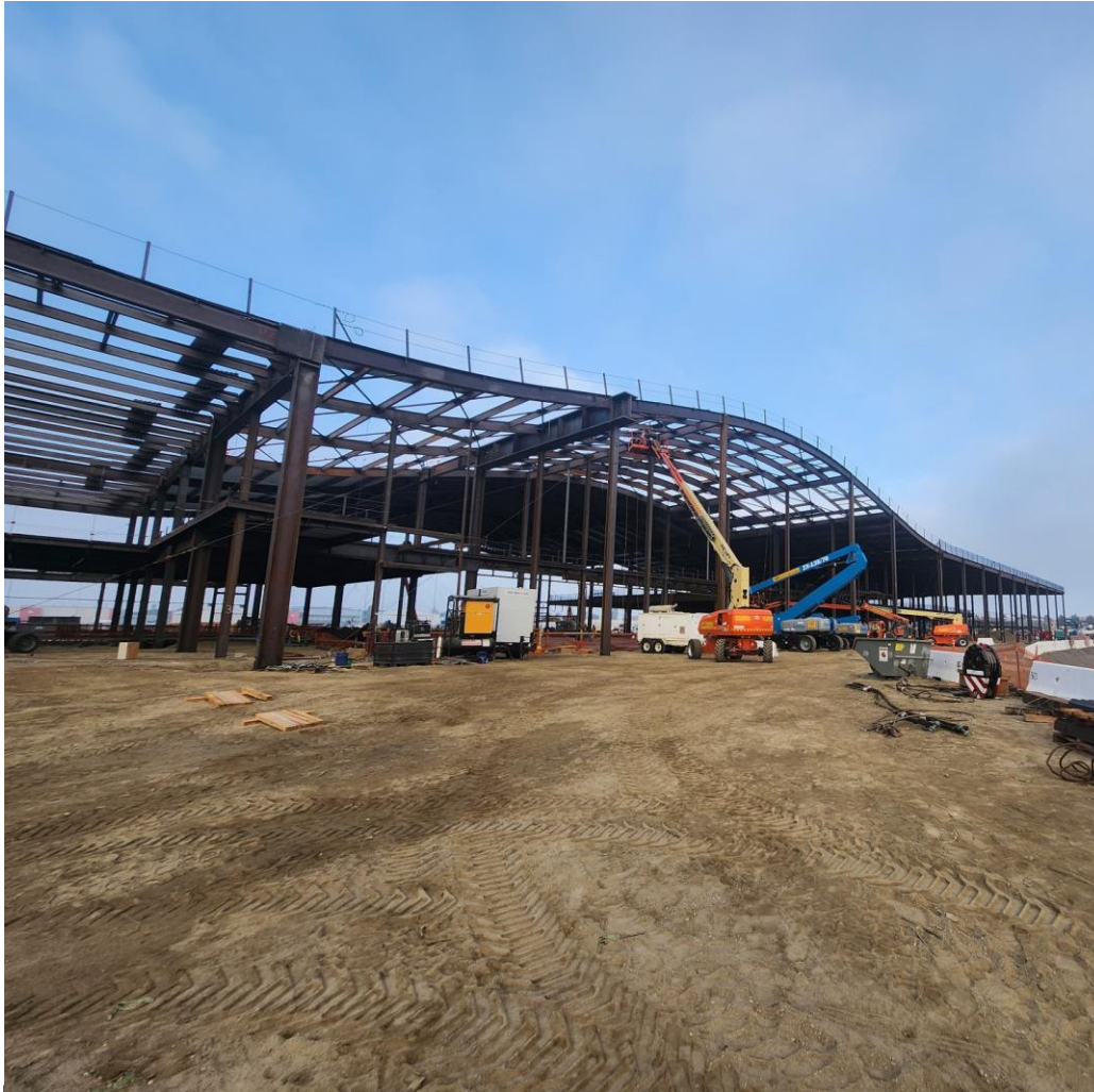
Terminal Area C Steel Erection
