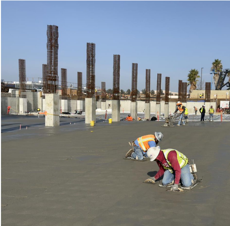
Parking Garage Slab Finishing
